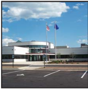
Water Treatment Plant Appleton, WI
